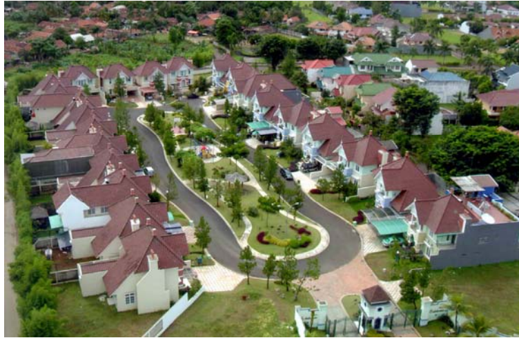
Figure 5: A Residential Cluster in BSD
